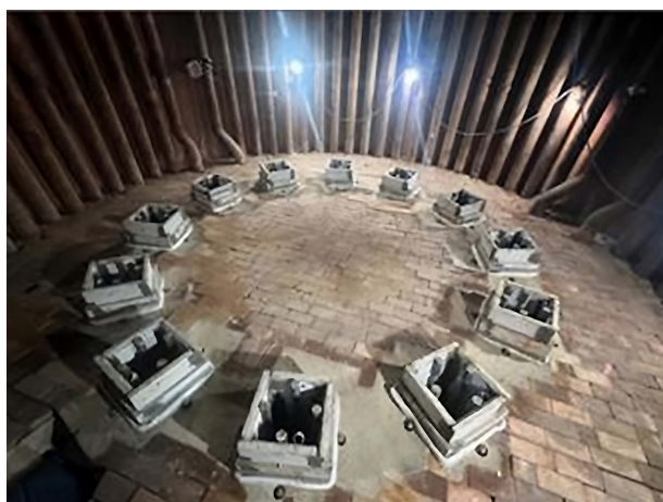
Figure 1. New burners installed in an operating unit.
